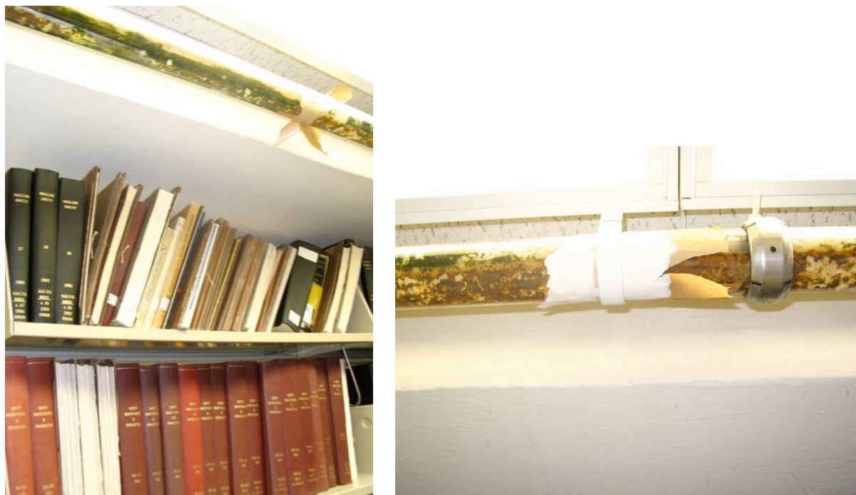
Figure 6: Exposed glass pipes with chemical waste
