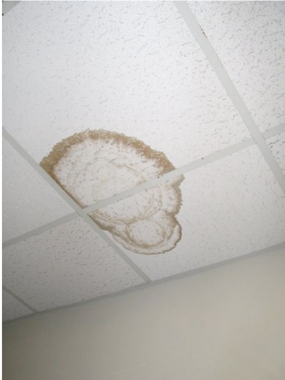
Figure 8: Damage from leaks in upper floor bathrooms
